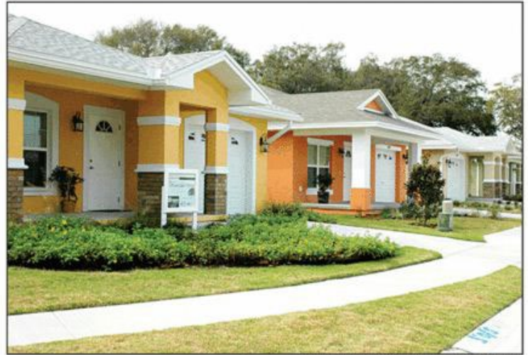
Photo courtesy of HABITAT FOR HUMANITY PINELLAS
